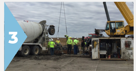
3 Foundation Drilling & Pouring
